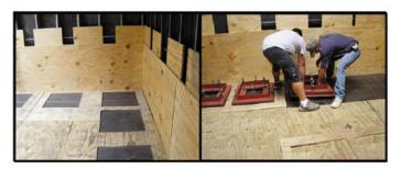
Here we are beginning the installation of a typical RD unit foundation. Plywood forms are used (supplied by Unisorb) to act as a template for the location of the individual RD units, and to provide a smooth surface on which to seal the concrete forms. This plywood is secured to the foundation block, and is lifted clear of the sub-slab when the foundation is raised into operating position. The RD Anchor Rings are then placed into the openings in the plywood.
