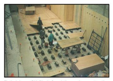
Typical large GK Block foundation under construction. Notice that the workmen are placing the plywood decking that in this case will support the concrete foundation.
