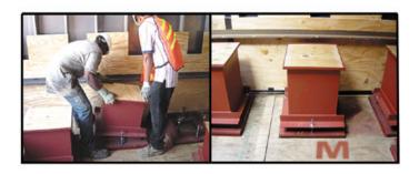
The adjustable length upper tubes are being installed. The finished upper level of the foundation is at the top of the RD unit.
