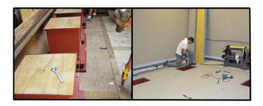
On the left the alignment process is shown as the RD units are brought into final position before the placement of reinforcing bars and the concrete pour.
