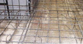
Pour the foundation utilizing proper concrete techniques. Be careful that the concrete flow does not push the rebar cage up tight against any of the IB-500-S2 sidewall materials.
