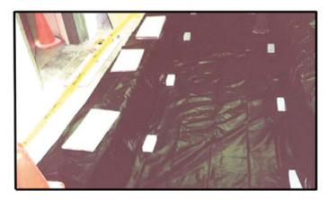
Here we have another view of the same foundation ready for the placement of the reinforcing steel and concrete.
