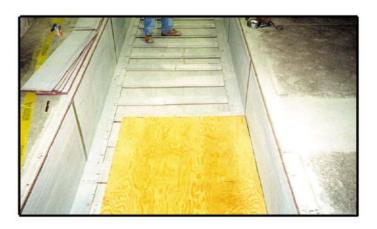
Here a mud mat is poured, then IB-500-B1 base material is applied in strips to achieve the desired pad loadings. In the foreground a sheet of treated plywood is being installed to protect the integrity of the spaces between the strips of base material (to prevent fluid concrete from entering the spaces). Notice that there is a strip of IB-500-B1 material around the perimeter of the base of the foundation as well as across (the full length).
