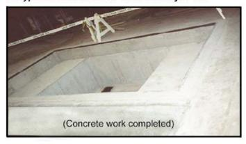
In this instance a concrete lined pit has been prepared due to less than ideal soil conditions. Note the "stepped" construction to establish the desired machine height.
