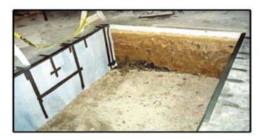
Note the exposed soil of the sidewall in this photo. Soil conditions at this location permitted a straight, smooth sidewall to be dug with minimal effort. Also note that the sidewall materials are taped to the concrete floor surface to hold them in place.
