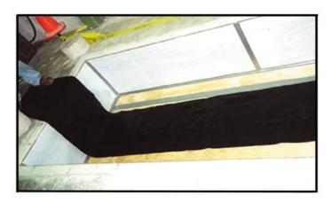
In this photo a Unisorb Poly Pit Liner is being installed over the treated plywood sheeting.
