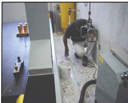
11. Application of Joint Filler V-100 Epoxy
