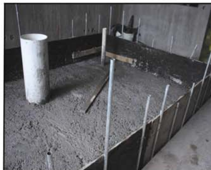
8. Inertia block concrete placed
