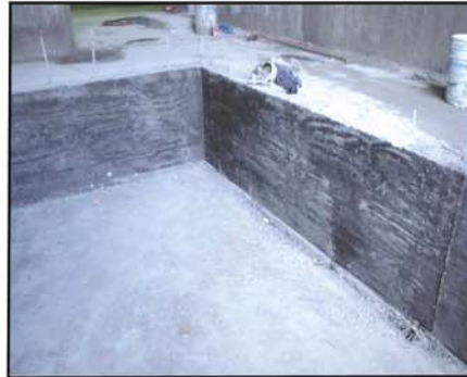
2. Concrete pit vault ready to receive UNISORB Foundation Isolation System
