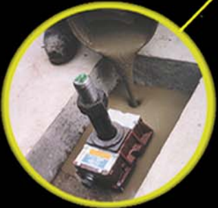
Advanced Grouting Techniques
