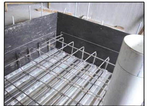
6. Reinforcing rebar cage
