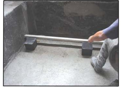
3. Placement of UNISORB GK Foundation Isolation Blocks
