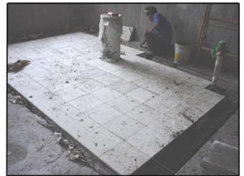
9. Granite tile installed
