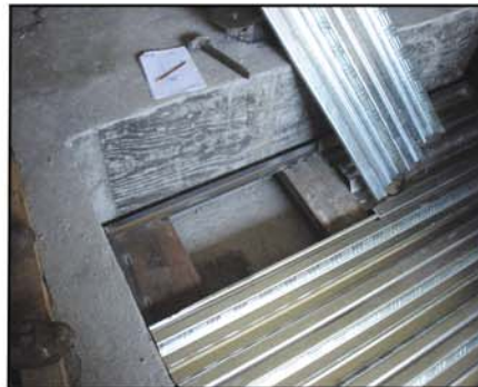
5. Setting of underlayment decking to support foundation
